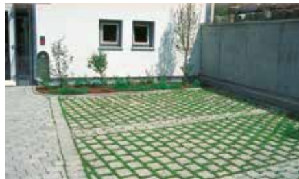
Pavement joint greening
