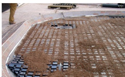
The drainage element Floradrain® FD 60 provides sufficient water retention capacity and made the old permanent irrigation system superfluous.
