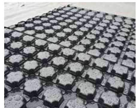
RS 60 retention spacers were used on all green roofs providing retention space below the wildflower/sedum build-up. All pictures ©Pritchard & Pritchard Ltd.
