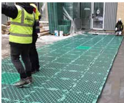
The heavy duty RSX spacers were laid on all podiums allowing them to be used as roof gardens with hard and soft landscaping.
