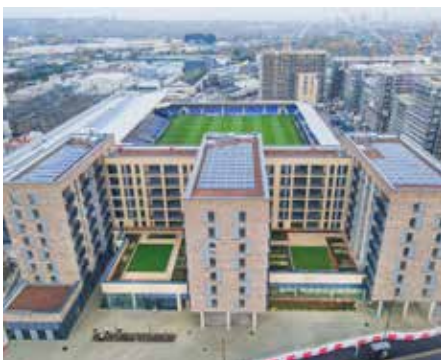
The huge mixed-use development at Wimbledon Grounds including vast 15,967 sqm area of ‘blue’ roofs and ‘blue’ podiums is one of the largest blue roofing projects in the UK.
