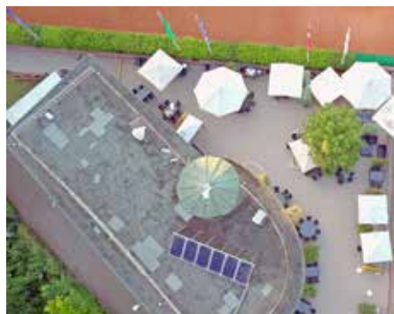
The KETV roof as a “naked” bituminous roof prior to the re-design as a green roof.
