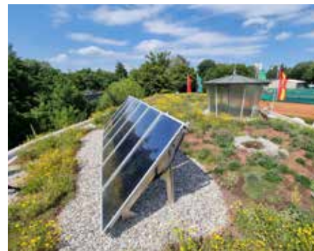
The green roof was combined with the existing solar energy unit – therefore producing synergy effects.
