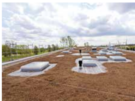
The pre-loaded system substrate "Rockery Type Plants".
