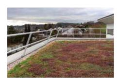
A collective fall protection solution such as Fallnet® ASG has the advantage that each person working on the roof is at the same time protected from falling off the roof. The ASG Maintenance Guardrail can be installed either vertically or at an angle. The Fallnet® ASG is Dekra-certified.
