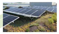
For an assembly of type "Butterfly", the two Solar Base Frames meet with their lower sides. Rainwater is directed to the middle of the Solar Base SB 200 and
