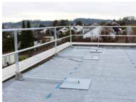
The post modules before the green roof system build-up is installed.
