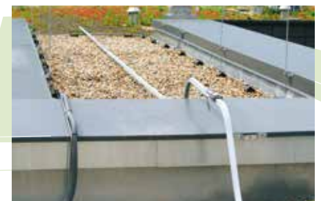
An s-shaped rail element elegantly addresses the changing height, allowing the runner to continue gliding without obstruction.
