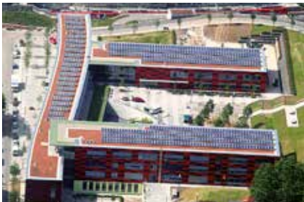
Solar energy systems are often installed right out to the roof edge to fully utilise the roof areas.
