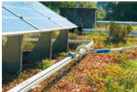
The fixing device in operation. The horizontal, gliding runner for personal protective equipment provides for maximum user friendliness.
