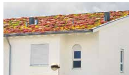
A shear barrier is placed just above the eaves on this monopitch roof, which is drained by means of an outer-lying gutter.
