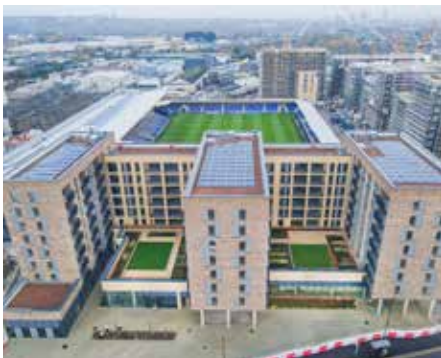
The huge mixed-use development at Wimbledon Grounds including vast 15,967 sqm area of ‘blue’ roofs and ‘blue’ podiums is one of the largest blue roofing projects in the UK.
