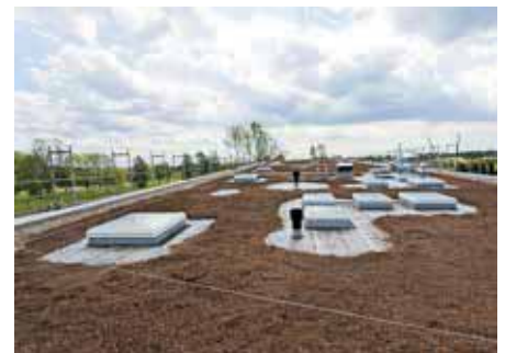
Installed system substrate "Rockery Type Plants".
